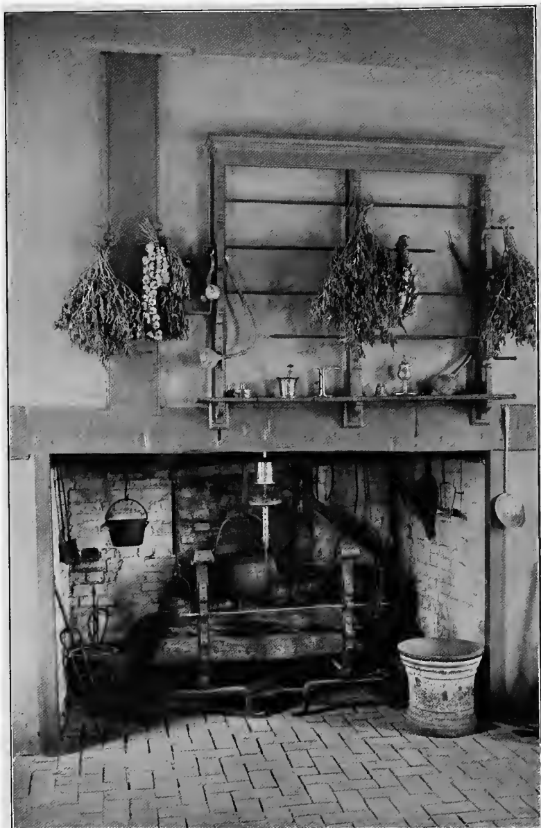
THE KITCHEN FIREPLACE
